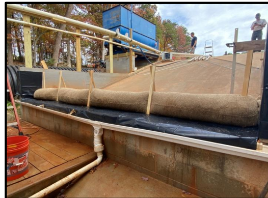
Typical Test Setup and SRD Installation
